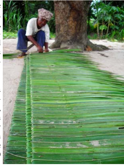
Mama Mbadgina of Yoyo village makes thatched roofing for the hotel redecoration.
